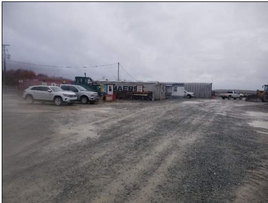
Figure 12-2: Core logging (grey trailer on right) and core cutting facilities (red trailer on left)
