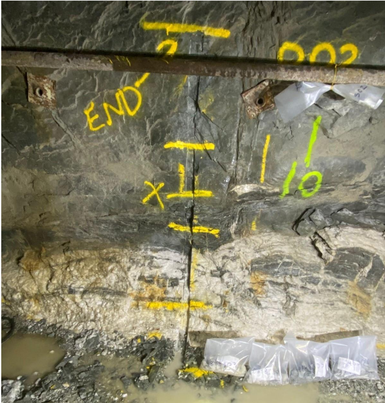
Figure 6: Channel sampling of the visible limbs in the floor of the drift at the 940 Level, underground at the Aureus East Gold Project.
